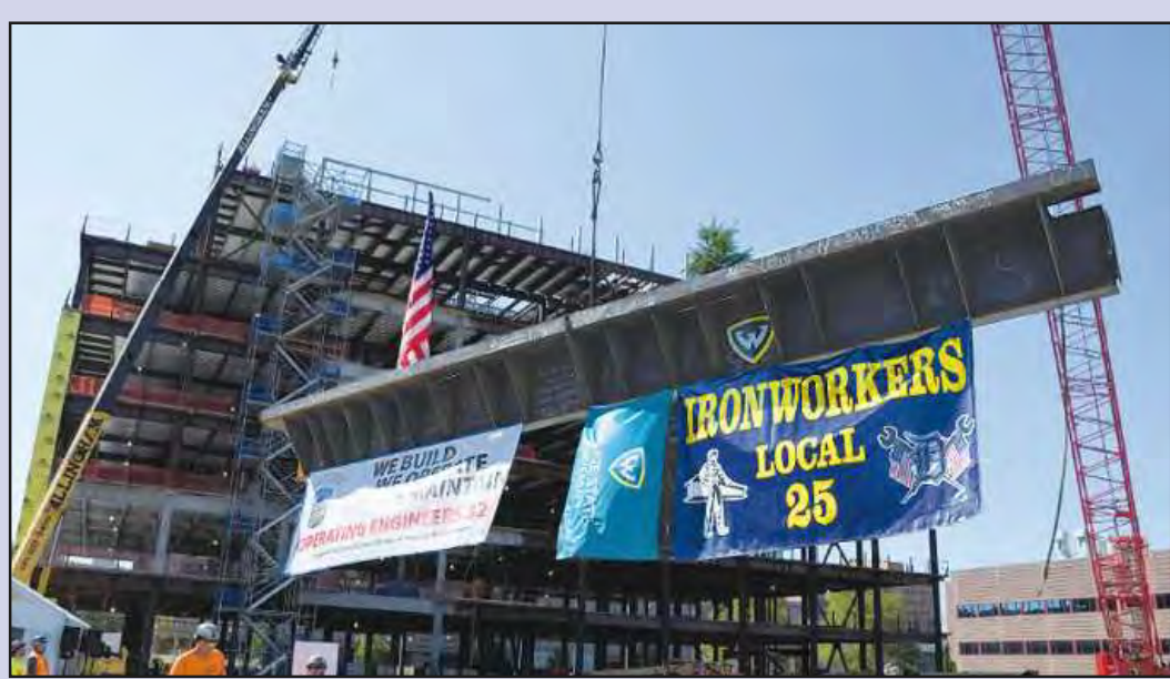
THE HEALTH SCIENCES Research Building on Wayne State University's campus was topped out Aug. 4, about a year after construction began on the $200 million project. Ideal Steel has been erecting the steel, and Christman Construction has managed the entire project.
