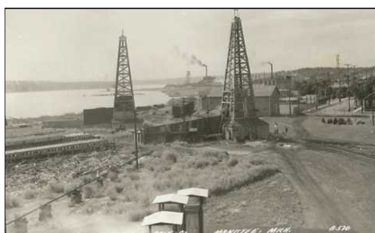
BRINE EXTRACTION WELLS are prominent in this 1930 view of the Morton Salt Co. plant in Manistee. Operators would inject water into the ground, forcing up salt, which was allowed to dry on the surface. That wet process is different from the dry extraction method of the salt mine under Detroit, which is taken out in the form of salt crystals. Morton Salt invented the retail packaging of salt, as well as the Morton Salt girl, and the slogan "When it rains it pours."
