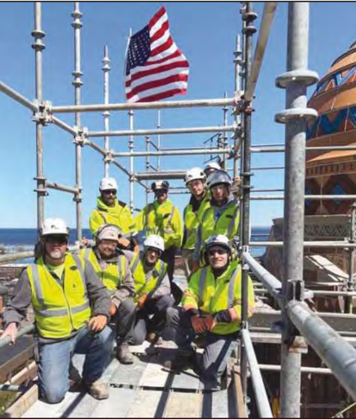
GATHERING FOR A PHOTO on the scaffold at the St. Peter Cathedral project are (l-r) RAM Foreman Bill Klein, bricklayer Robert Barrett, laborer Dennis Emanuelson, bricklayer Shawn Pietila, bricklayer Chris McCormick, bricklayer John O’Connor, laborer Daniel Flynn, laborer Shane Cromell, bricklayer Lucas Flygare and not pictured bricklayers Antwan Stone and Brian Lantto.
