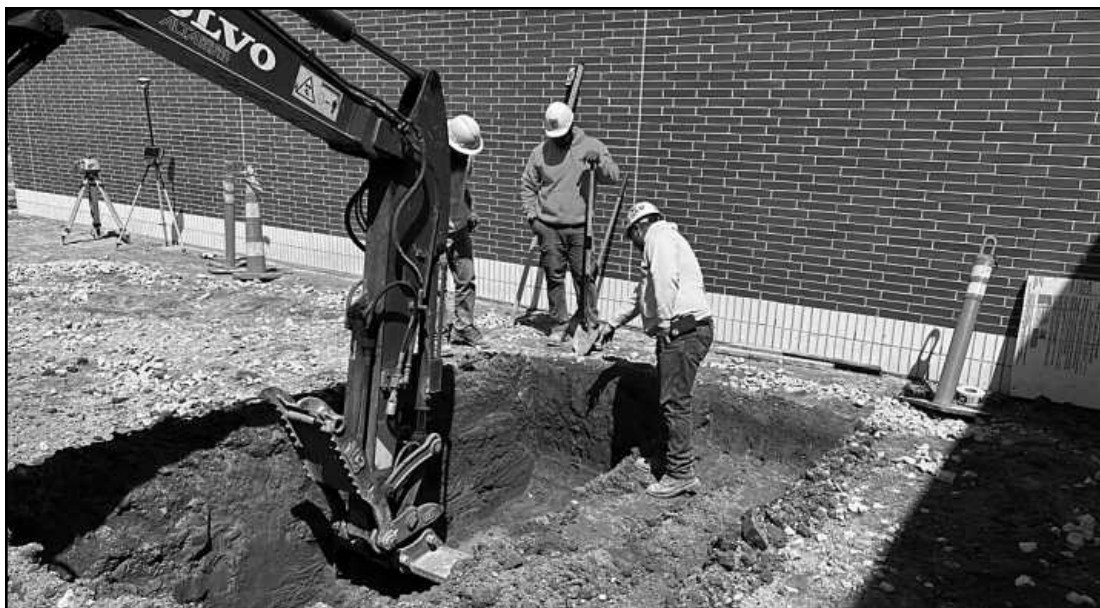
DIGGING THE FOOTINGS for an above-ground fuel tank at the Northville Twp. psychiatric hospital site are (l-r) Laborers Ethan Warren (Local 499), Walter Johnson (Local 499) and Jim Barr (Local 1191). They're employed by Site Development.
