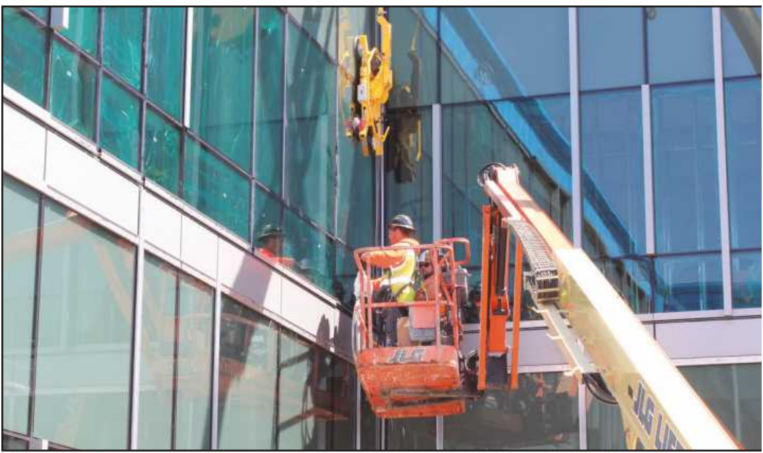
SETTING WINDOWS at the Northville Twp. psychiatric hospital project are Garrett Fowler and Jacob Tyslicki. The Glaziers and Glassworkers Local 357 members are employed by Edwards Glass.
