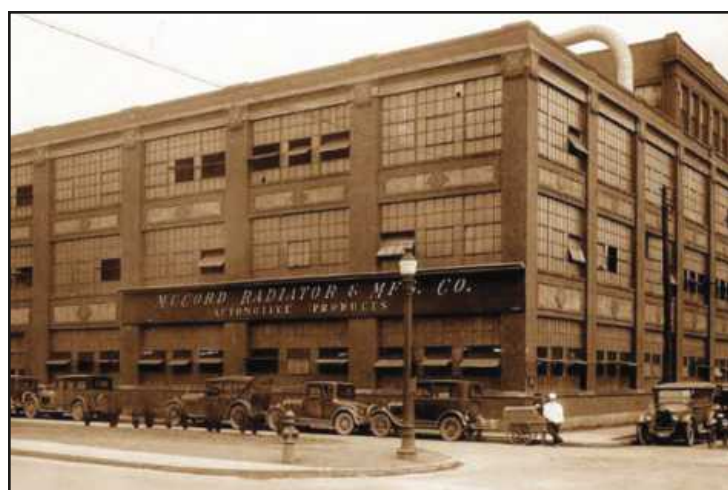
PART OF THE MCCORD Radiator and Manufacturing Co. factory at 2587 East Grand Blvd. in Detroit, in 1935. During World War II, plant workers there produced 20 million M-1 steel helmets.
