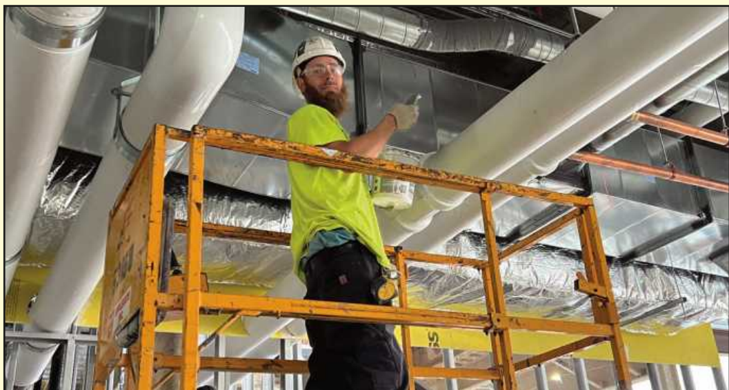
GIVING US A LOOK at his brush work as he seals a duct at the new Lansing Public Safety headquarters is Traye Worden of Sheet Metal Workers Local 7. He's employed by Applegate.
