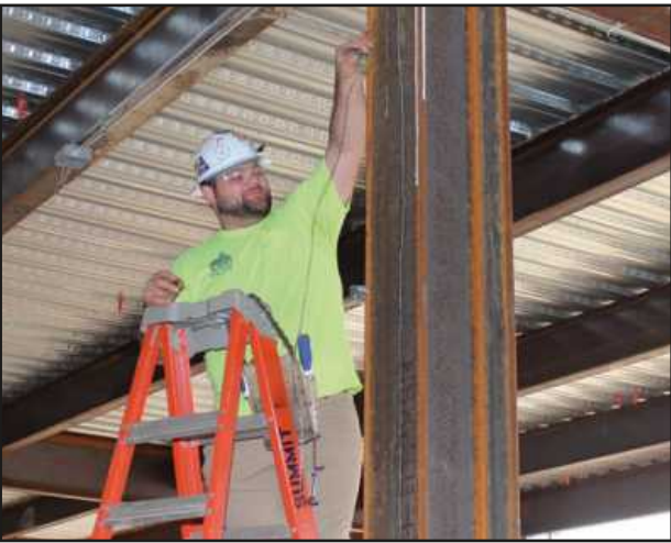
FITTING A PIECE OF CONDUIT on the first level of the Lansing Public Safety Building is Braedon Riggs of IBEW Local 665. He's employed by Summit Electric.
