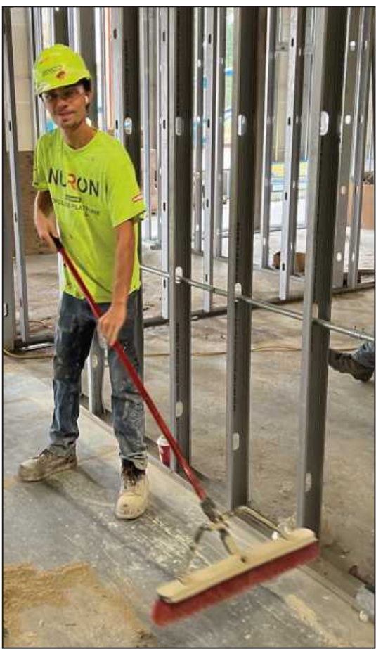
A CLEAN SWEEP on a second level hallway at the Lansing Public Safety project is made by Caleb Ricketts of Laborers Local 1191. He's employed by William Reichenbach Co.
