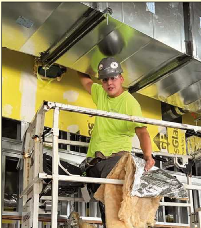
INSULATING A DUCT at the Lansing Public Safety Building project is Landen Heller of Heat and Frost Insulators Local 47. He's employed by Bondy Insulation.
