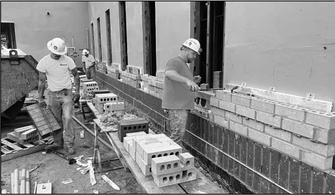
SETTING A BRICK COURSE on an exterior wall at the new fire station on the Lansing Public Safety campus are (l-r) laborer Caleb Barnett (Local 1075) and masons Jason Chrysler and Lucas Grubaugh (Bricklayers and Allied Craftworkers Local 2). They’re employed by Davenport Masonry.
