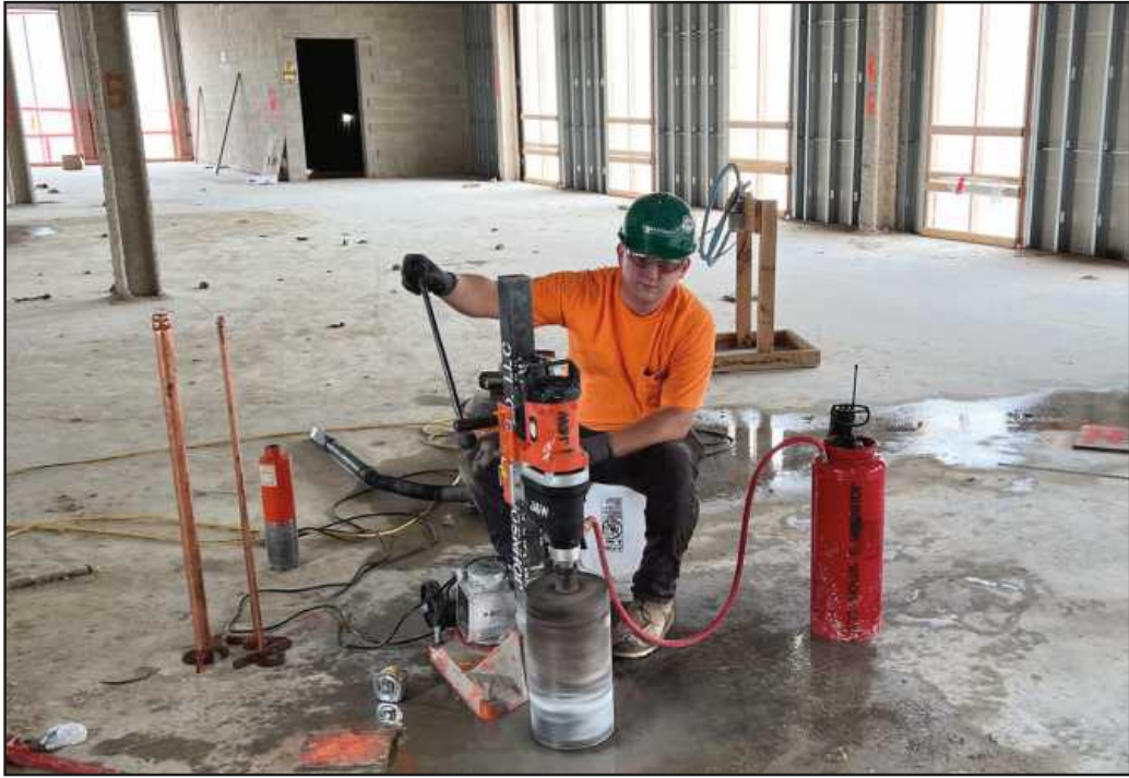
CORE DRILLING for a pipe between floors at the Lansing Public Safety building project is Kyle McKibben of Plumbers and Pipe Fitters Local 333. He's employed by Johnson and Wood.
