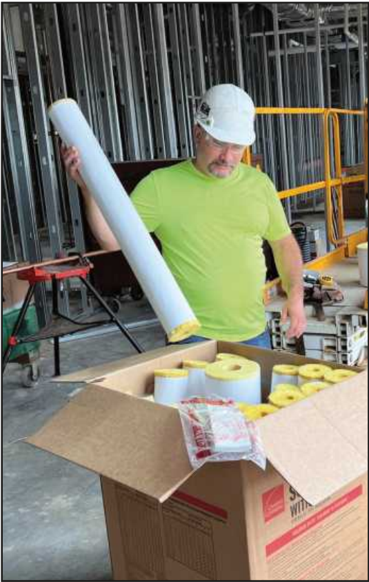
SELECTING A SECTION of pipe insulation for placement on the second level of the Lansing Public Safety Building project in Lansing is Chris Pangborn of Healt and Frost Insulators Local 47. He's employed by Bondy Insulation.
