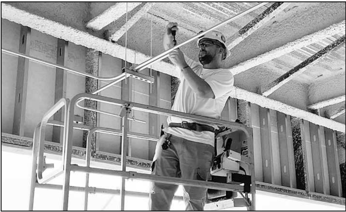
RUNNING CONDUIT in the ceiling of the second level of the new Lansing Public Safety Building is third-year apprentice Chris Allen of IBEW Local 665. He’s employed by Summit Electric.
