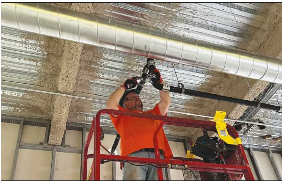
SETTING A VENT PIPE CONNECTION while working at the Lansing Public Safety Building is Ted Westbrook of Plumbers and Pipe Fitters Local 333. He’s employed by Johnson and Wood.
