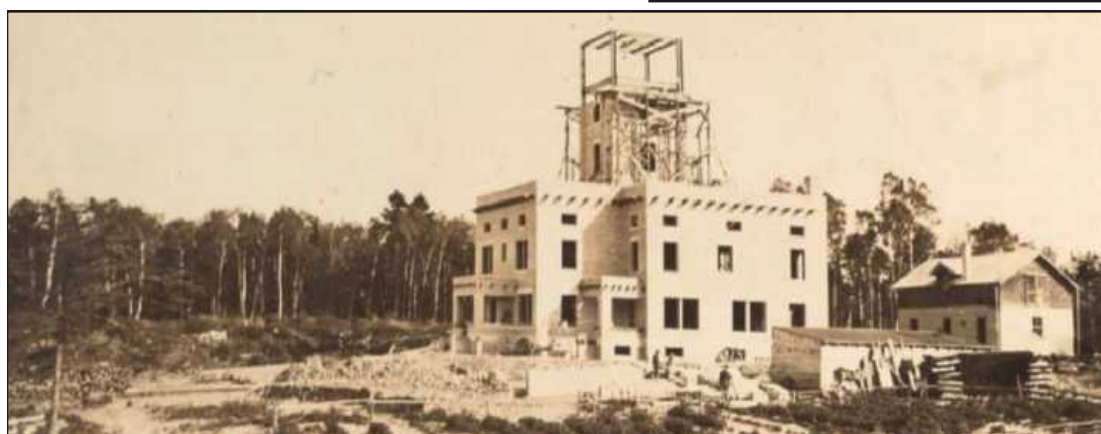
THE SAND HILLS LIGHTHOUSE under construction in Ahmeek in the Keweenaw Peninsula in September 1918. Its first light would shine in June 1919. Photo credit: Lighthouse Friends
