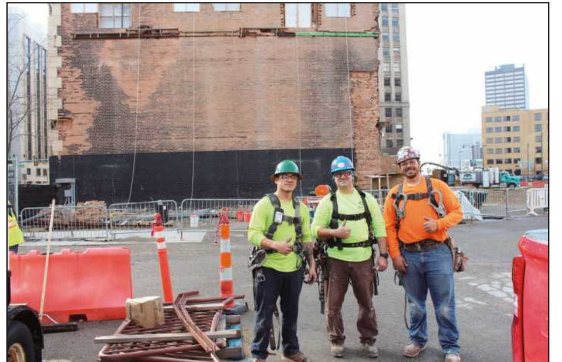
YOU WANT A SOLID PLATFORM? Scaffold erectors on the grounds of the 150 Bagley project in Detroit include (l-r) Noah Morales, Rick Baumia and Justin Guthrie. The Michigan Regional Carpenters Council Local 687 members are employed by... Solid Platforms.
