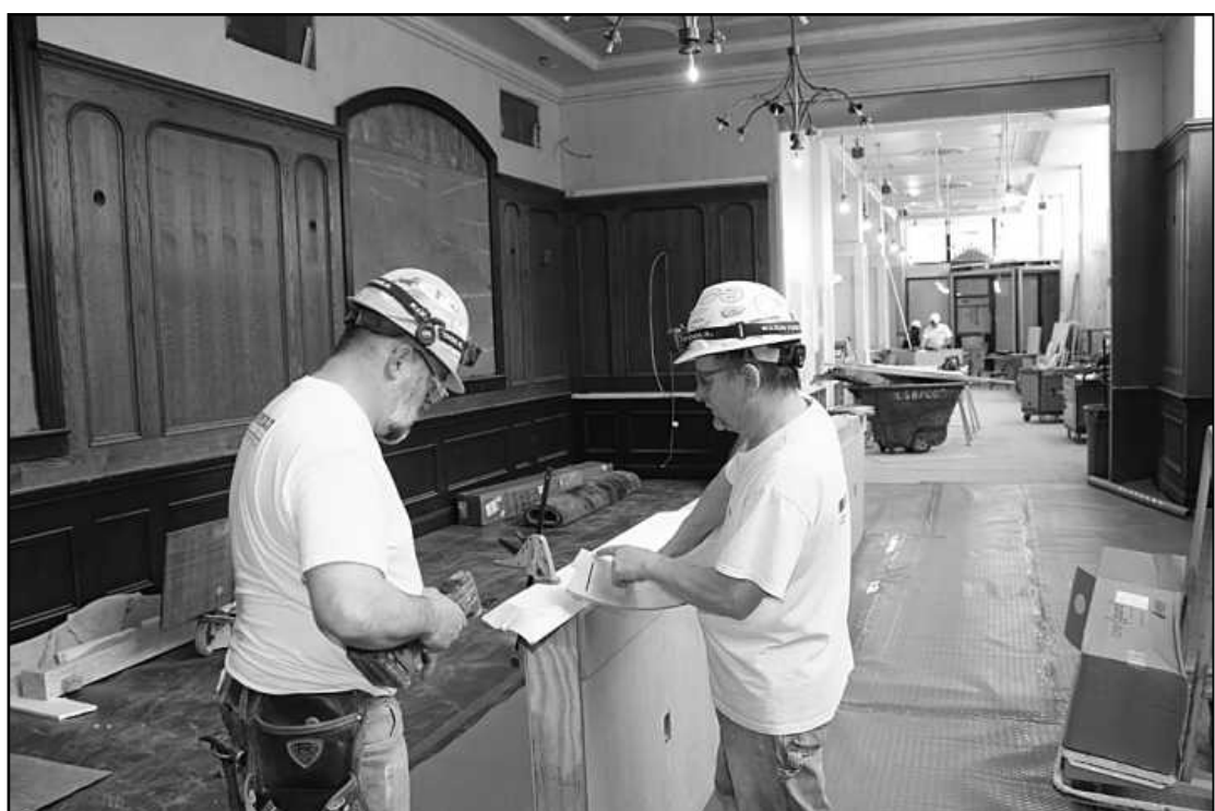
SHAVING SOME CROWN molding in what will be first floor restaurant space of the Book Tower project in Detroit are John Schleben and Chris Hinkle of Michigan Regional Carpenters Council Local 687. They're employed by Christman Constructors.
