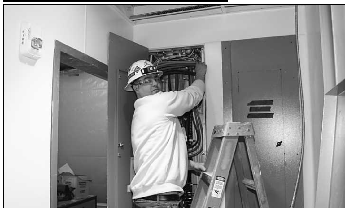
ELECTRICIAN Kamil Chanski of IBEW Local 58 wires a first floor lighting panel at the Book Tower project in Detroit. He's employed by Edgewood Electric.
