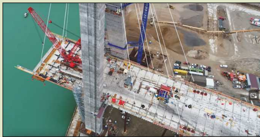
THE BRIDGE DECK is starting to extend over the Detroit River toward Windsor, Ontario. The construction process continuously extends single-deck segments before meeting in the middle of the Detroit River with the Canadian span.
