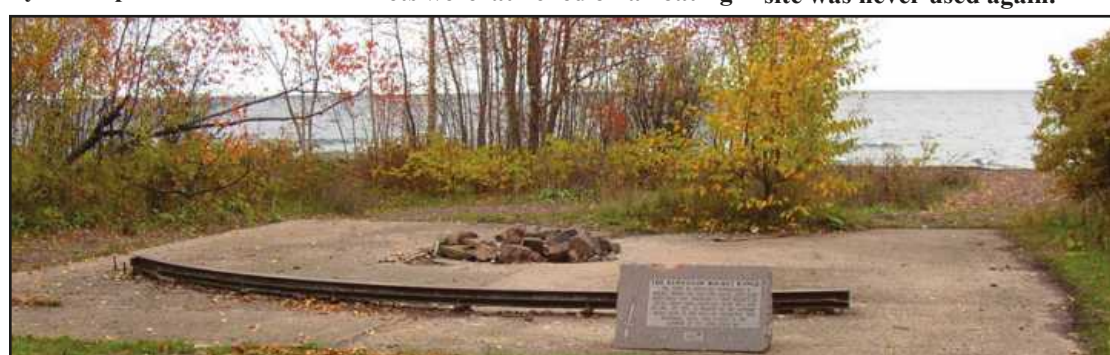
WHAT’S LEFT OF THE KEWEENAW Rocket Range today – not much, just the concrete launching pad and a stone monument marking what took place there from 1964-1971 on the Lake Superior shore. “In tribute to the historic work done in the field of rocketry” says an inscription on the monument, which was placed in 2000. The steel set in the concrete was an “azimuth ring,” used for aiming the rockets.
