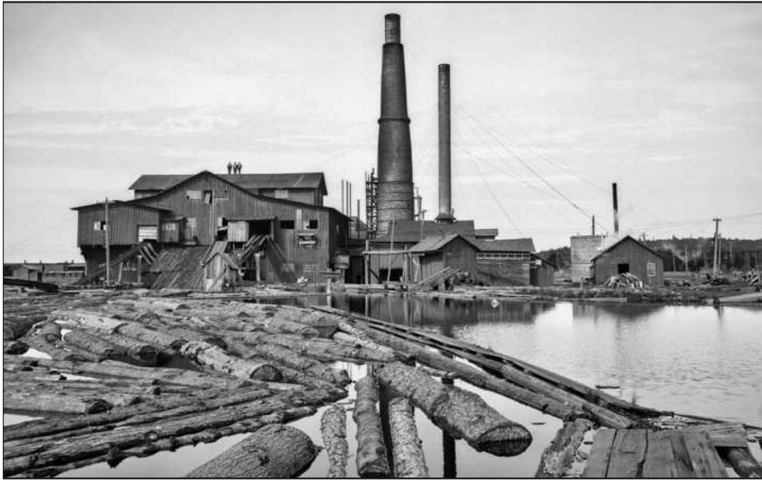
THE SAWMILL at the mouth of the Dead River in Marquette, in 1905. Sawmills were usually sited at the mouth of Michigan rivers, allowing logs to be floated in their direction. The timber would then be cut, bundled and moved by railroad or ship to other Great Lakes ports. Mill workers were paid more than forest-based loggers, but had to pay their own room and board. Changes in lumber-cutting technology drove major efficiencies. In the 1860s steam power came into play, and by the end of the 1870s virtually every mill operation had been mechanized to some degree, according to Lumbering in Michigan . The first circular saws of the 1860s had wide, wobbly blades, producing miles of sawdust. Thinner blades soon arrived, then bandsaws, which eliminated the poorer quality cuts of their predecessors.
