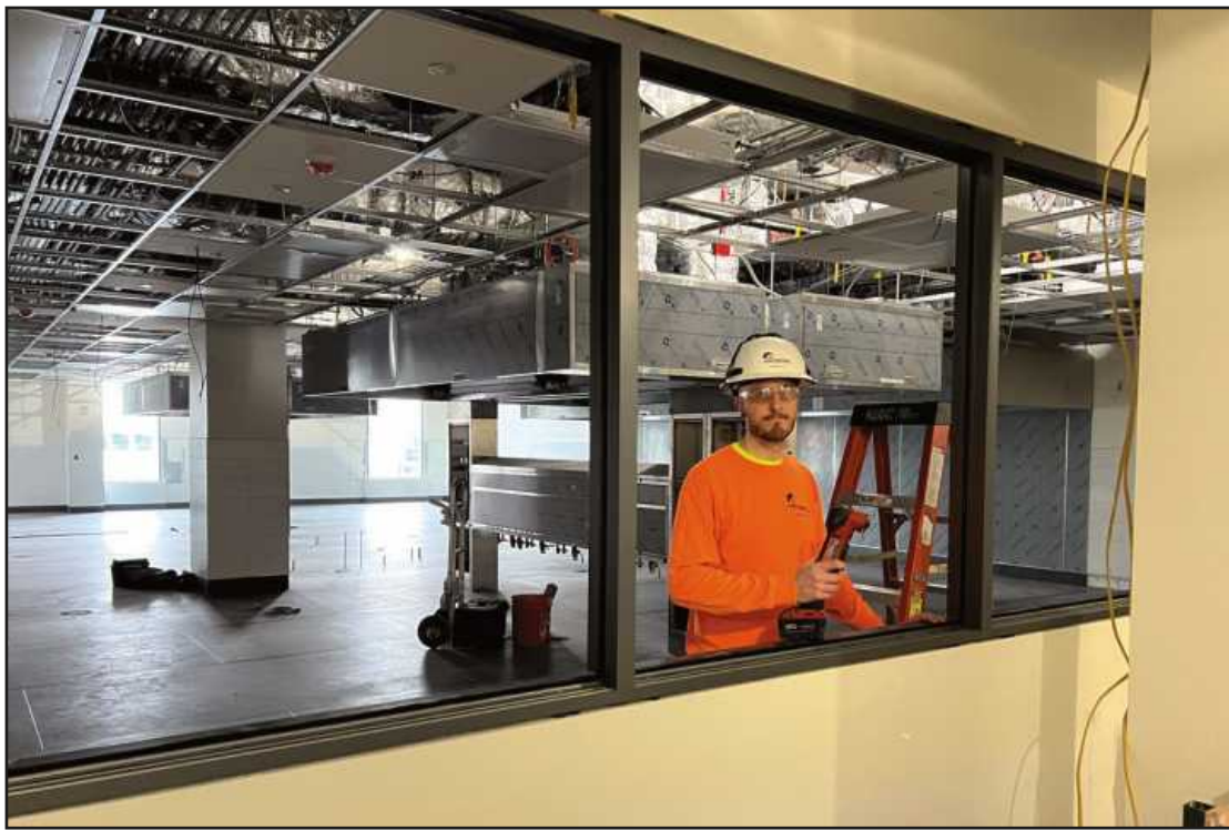
INSTALLING A "STOREFRONT" hallway window that looks into kitchen space at the Oakland Community College Culinary School project in Royal Oak is Devon Stepp of Glaziers and Glassworkers Local 357. He's employed by Universal Glass.
