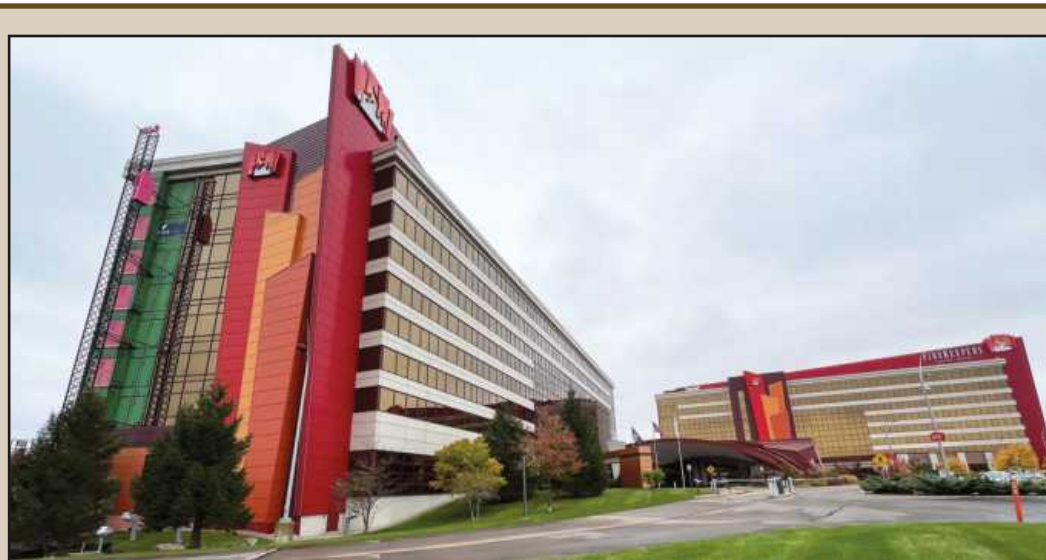
ONE OF THE TWO HOTEL towers, left, at the Firekeepers Casino is undergoing a major "refresh" of its interior rooms. In an effort led by Clark Construction and mechanical contractor Andy J. Egan, all of the tower's 243 rooms are being renovated. A buck hoist attached to the tower, at left, provides the trades with easier access to the rooms.
