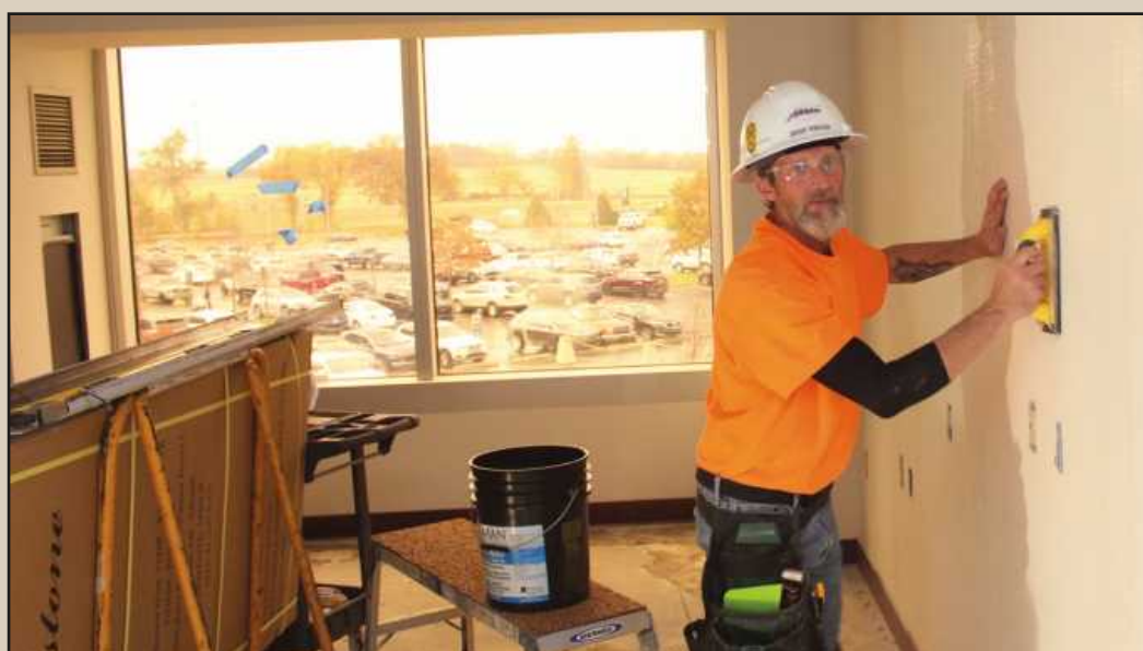
SANDING DRYWALL in a second-floor guest room that's getting refurbished at Firekeepers Hotel in Battle Creek is Jeremy Vergeson of Michigan Painters District Council 1M- Local 845. He's employed by Murray Painting.
