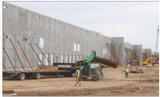
OFFLOADING RE-ROD for placement at the Amazon fulfillment center under construction in Delta Twp. are Iron Workers Local 25 rodbusters, employed by Fessler and Bowman.
