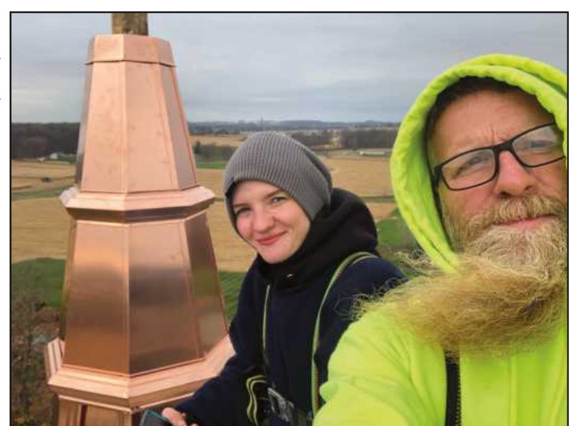
ERECTED IN 1908, St. Mary's Visitation Catholic Church in Byron Center now has a gleaming new steeple cover. The copper covering was primarily cut and installed by Sheet Metal Workers Local 7 foreman Brad Olson and his daughter, apprentice Hannah Berg.
