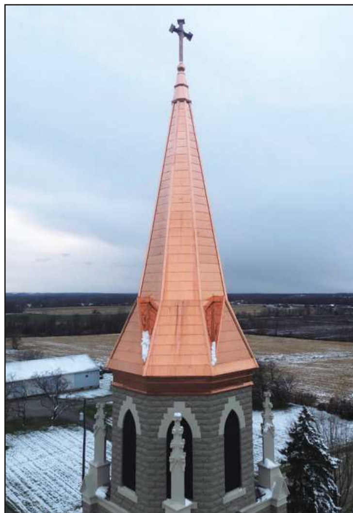
THE NEW COPPER-COVERED steeple above St. Mary's Visitation Church in Byron Center.
