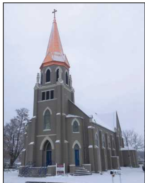
ERECTED IN 1908, St. Mary's Visitation Catholic Church in Byron Center now has a gleaming new steeple cover. The copper covering was primarily cut and installed by Sheet Metal Workers Local 7 foreman Brad Olson and his daughter, apprentice Hannah Berg.
