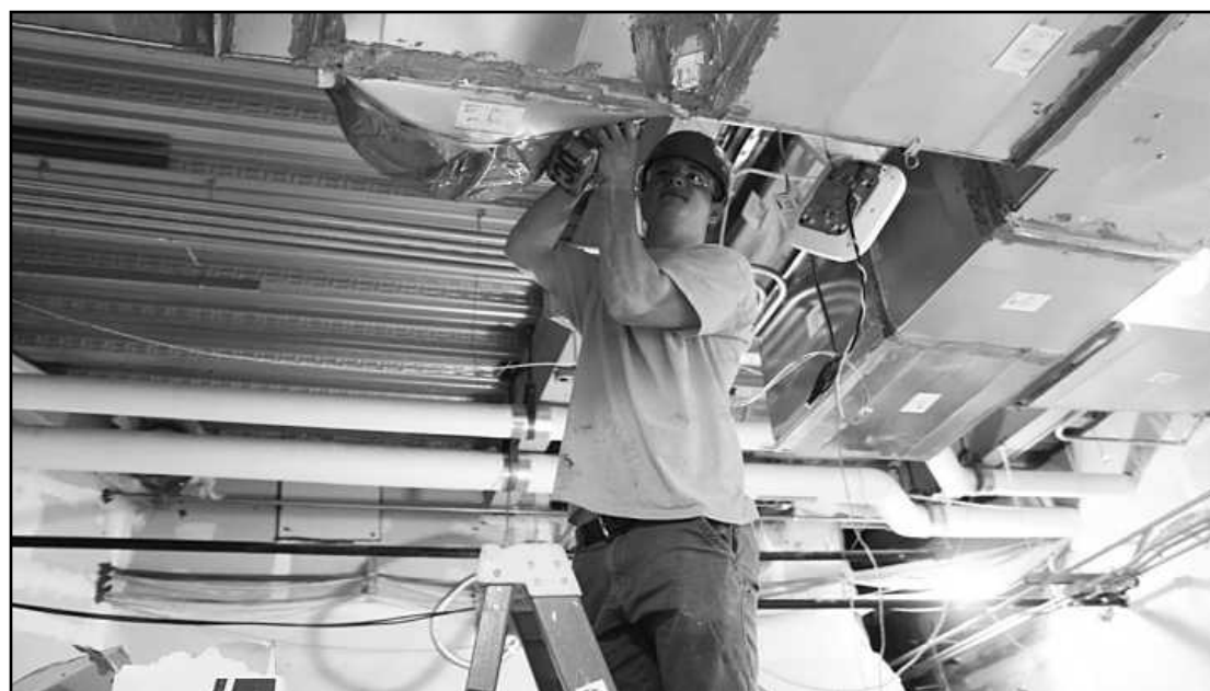
WORKING ON A SHOE TAP DUCT SECTION at the existing Trinity Health-Brighton hospital project is Dean Battley of SHEET METAL WORKERS LOCAL 7. He's employed by Dee Cramer.
