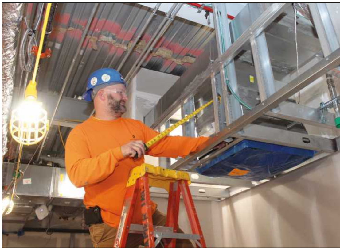
MEASURING FOR A SECTION of exhaust duct at the Trinity Health-Brighton hospital project is Clay Biggs of Sheet Metal Workers Local 7. He's employed by Dee Cramer.
