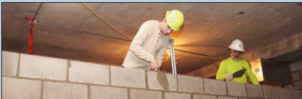
SETTING A BLOCK WALL in the basement of what will be the Genesee County Building are Matthew Ellis and Wilbur Cox of Bricklayers and Allied Craftworkers Local 2. They're employed by B & G Masonry Service.
