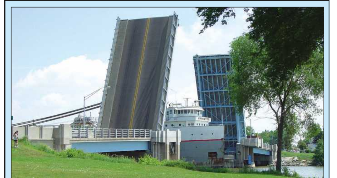
THE SOUTHERN MOST bridge along the Saginaw River in Bay City, the Lafayette Street Bridge has had a significant amount of repair and rehabilitation work since it was erected in 1938. “The bridge superstructure is continuous over the piers, an uncommon detail for a bridge of this type and age. With the exception of the original railings being replaced, the bridge retains excellent historic integrity,” says Historic Bridges. Photo credit: Wikipedia Commons
