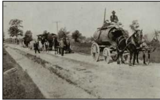
CONSTRUCTION MACHINERY for a macadam road in Saginaw County, 1905-06
