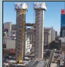
The building's pair of structural concrete spines.
