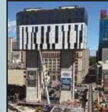
The building's 11th story was lifted in September.
