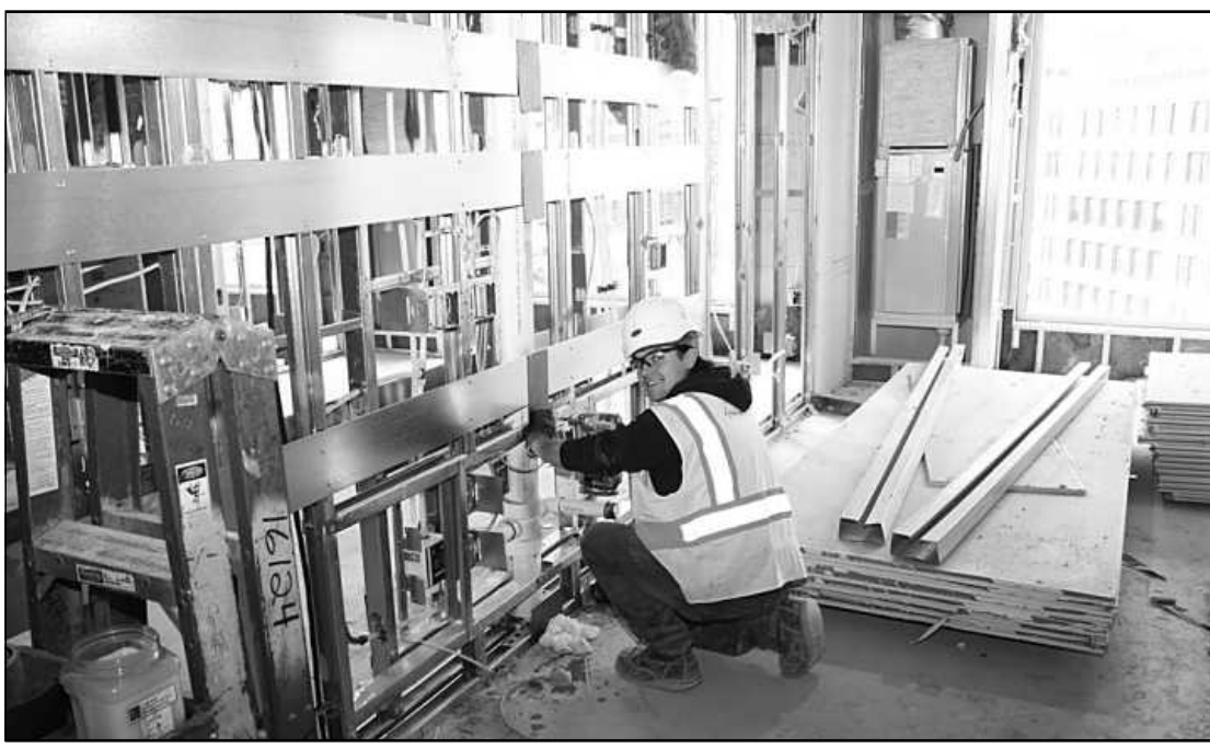
SETTING THE BACKING for plumbing fixtures in an apartment of the seventh floor of the Exchange Building in Detroit is Nathan Kopy of Plumbers 98. He's employed by Western Mechanical.
