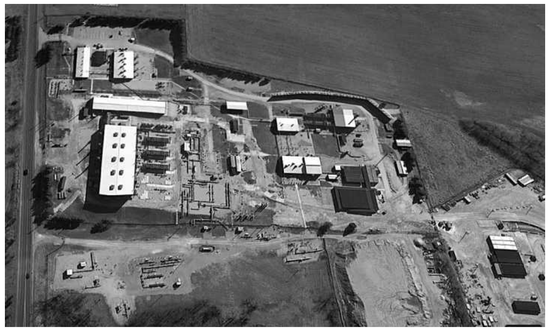
THE FREEDOM COMPRESSOR Station in Manchester.
