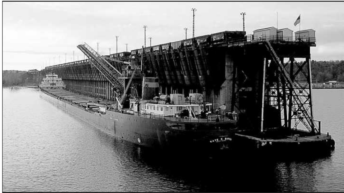
THE 767-FOOT-LONG freighter Kaye E Barker is shown lined up in a modern photo at the Presque Isle Ore Dock in Marquette, ready to accept gravity-fed iron ore pellets dumped from rail cars above. "Although the dock was originally built to load three ships on each side at once, its length allows it to accommodate the modern 1,000-foot vessels," said the Mining Journal . The ore dock is one of only three that are still operational in the upper Great Lakes.
