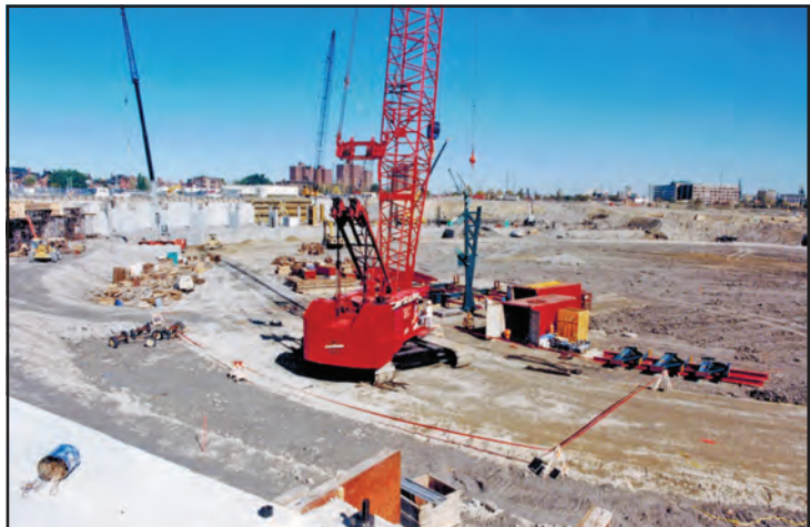
THE SETTING OF THE first column of iron.
