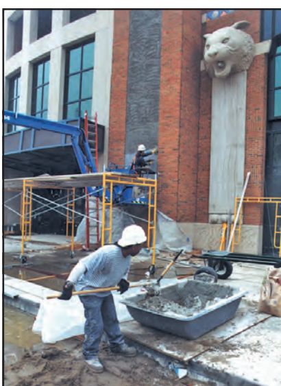
BAC Local 2 tile masons at work at Comerica Park.
