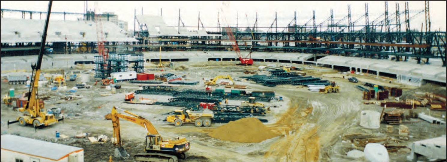
A PANORAMA OF the construction at Comerica Park.
